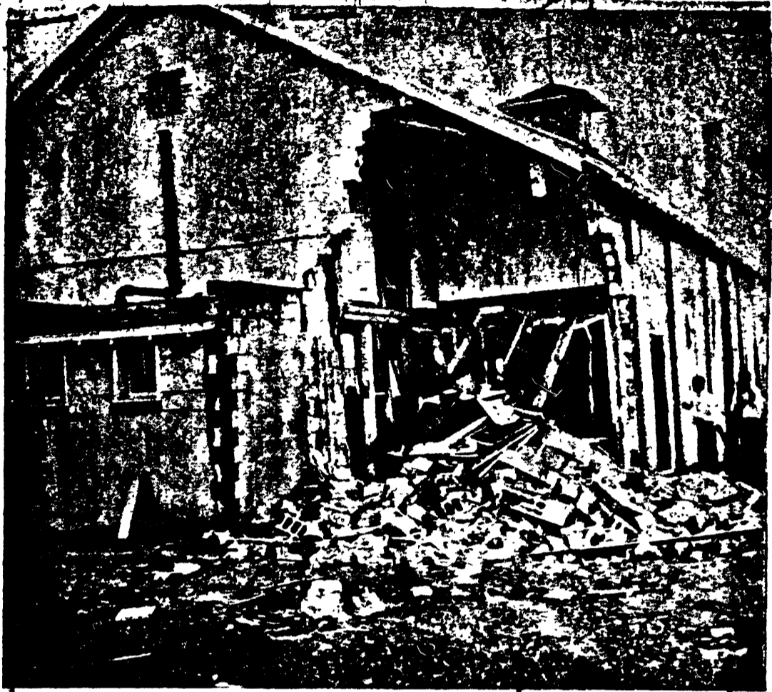
BELL STREET BAPTIST CHURCH CORNER DEMOLISHED All Windows In Church Shattered In Worst Explosion
