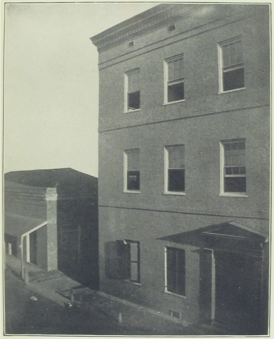
NO. 1.—TAKEN FROM THE BALCONY OF THE KING BUILDING, AND SHOWS THE REAR PORTION OF THE MILLER HOTEL FRONTING ON THIRTEENTH STREET.
