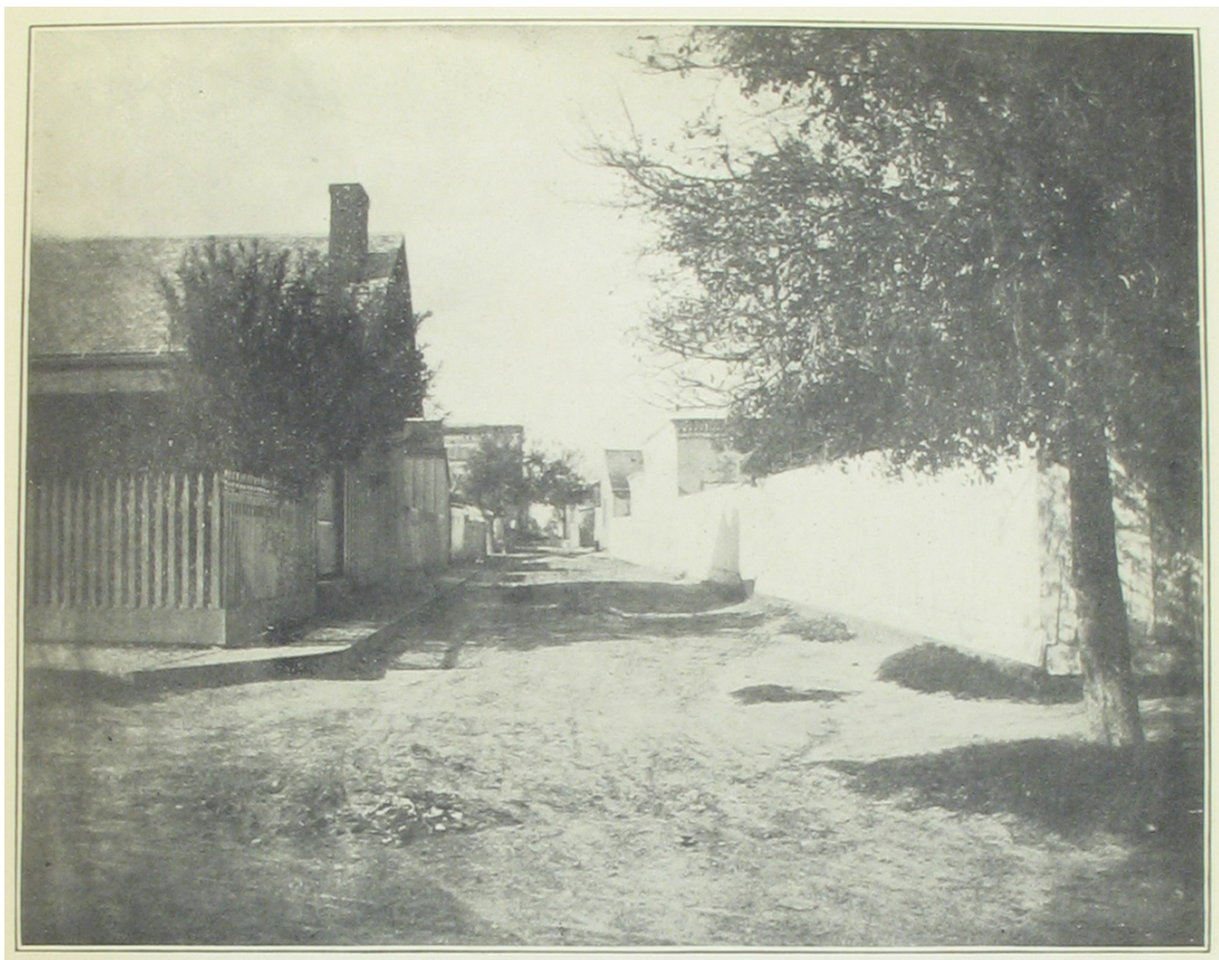
NO. 6.—TAKEN FROM GARRISON WALL, LOOKING NORTH UP THE ALLEY IN WHICH THE SHOOTING TOOK PLACE.
