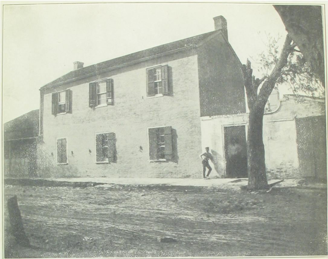
NO. 8.—REAR OF LEHY HOTEL. TAKEN FROM ALLEY AT SIDE OF COWEN HOUSE.
