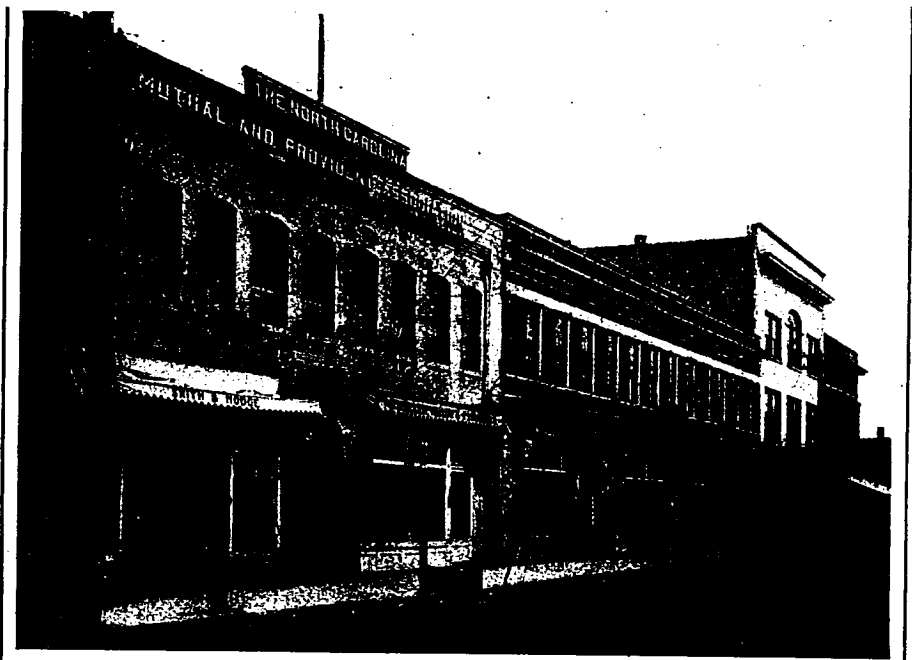
BUSINESS BLOCK OF THE NORTH CAROLINA MUTUAL AND PROVIDENT ASSOCIATION, AT DURHAM, N. C.
